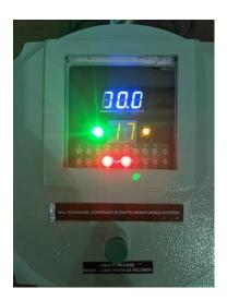
• Functions like HOLD, RELEASE, RESEST is also provided in the System for carrying out any repairs of earth faults, however it is not necessary to HOLD the circuit while repairing
